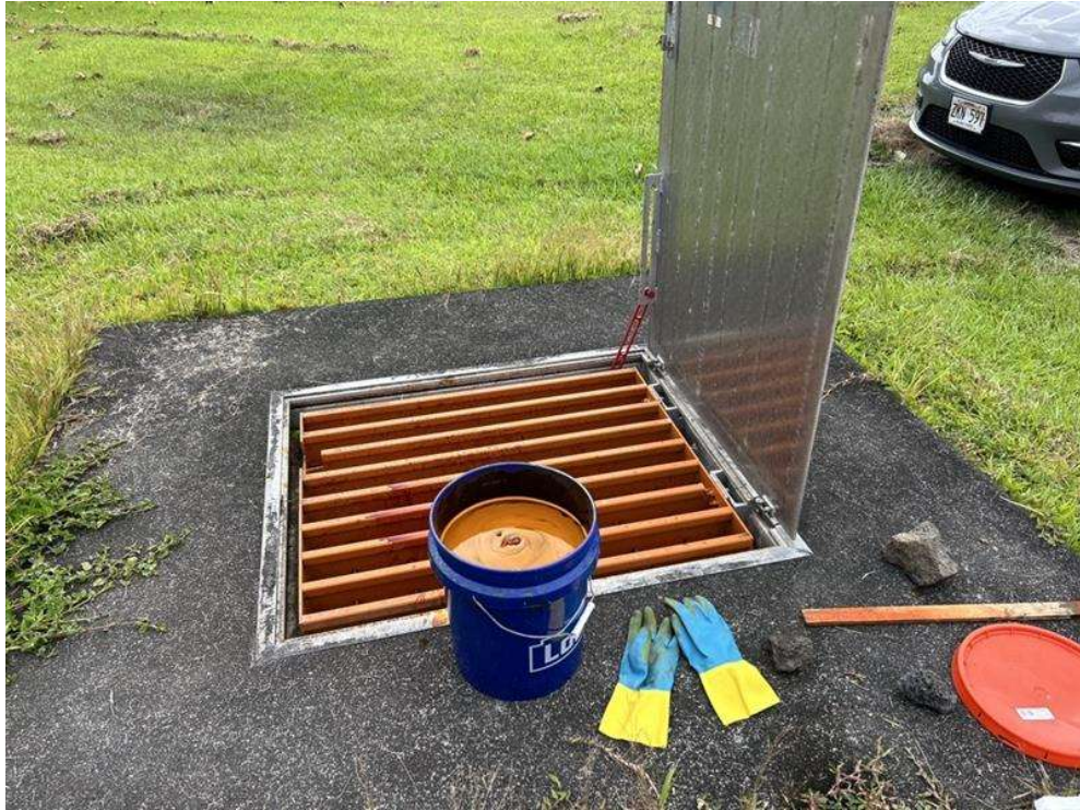
Figure 6. Manhole configuration (injection port) and dye setup for Hilo WWTP Outfall inspection
