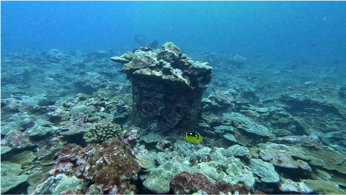
Figure 7. Manhole #4A, located at Station 44+63, shown with high coral cover and outfall pipe covered
