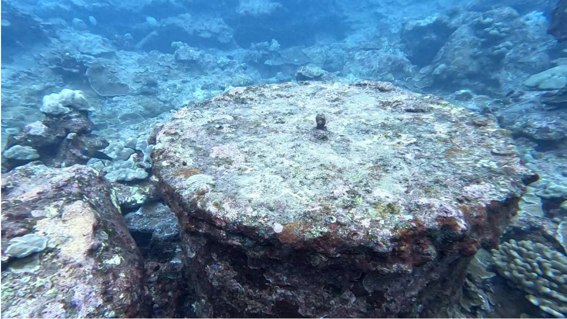
Figure 17. Manhole #2 located at Station 25+88 with no coral cover
